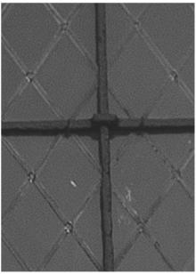
With the support of the Friends, and as part of the programme of repair recommended by the last Quinquennial Inspection, work has been completed on the windows of the tower of St. Mary's, redecorating their external ferrimenta (ironwork supporting the glass) and consolidating the clunch around the west window.
