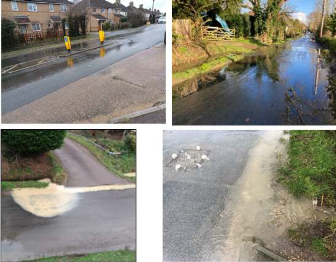
Figure 16. Photos demonstrating foul water flowing up through manhole covers on Swaynes Lane and Barton Road.
