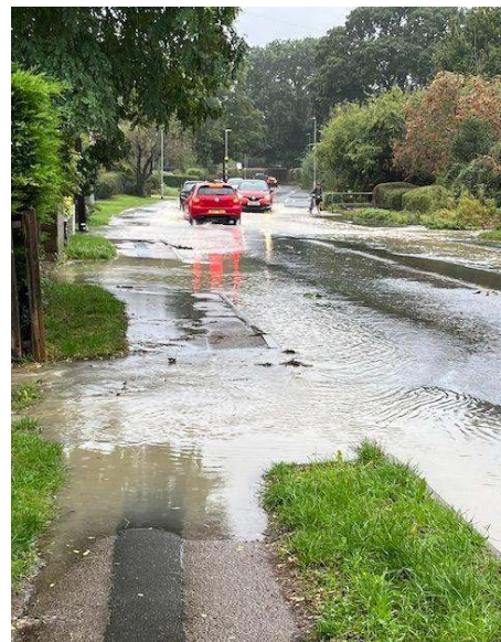
Figure 3 (right). Barton Road/Harbour Avenue Junction; several times a year at this level, mixed rainwater and Raw Sewage. Picture: 1st Oct 2024.
